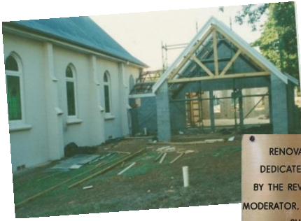
The Fellowship room taking shape.
