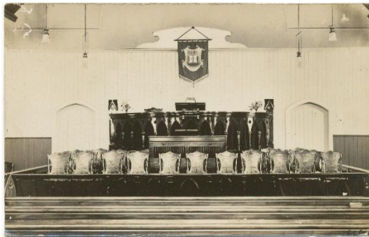
(Left) The original construction with the drop wall 1914/15
